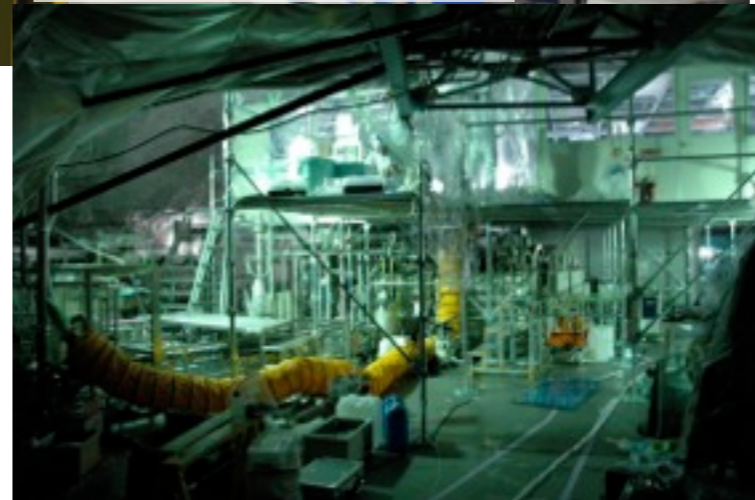
Clean room in the dome
