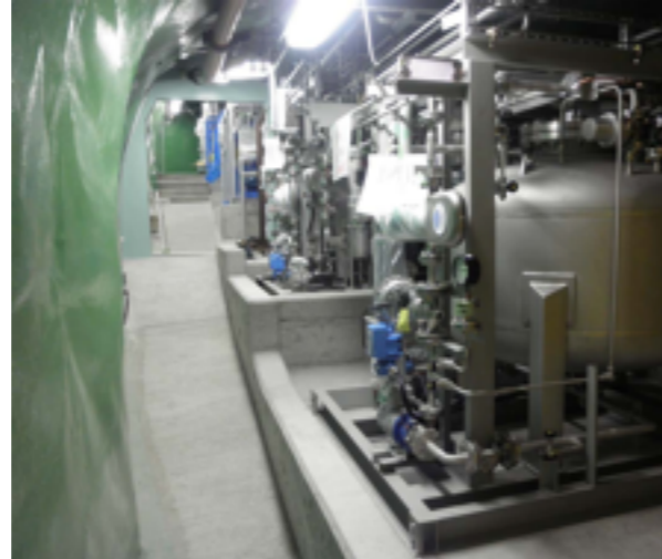
Xenon mixer and density control system
