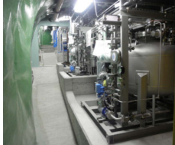
Xenon mixer and density control system
