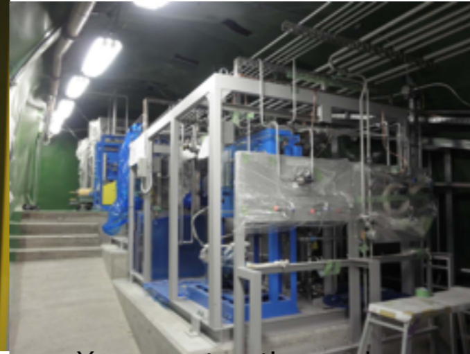
Xenon extraction and storage system
