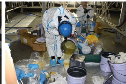
Mixing two materials (main and curing agent)
