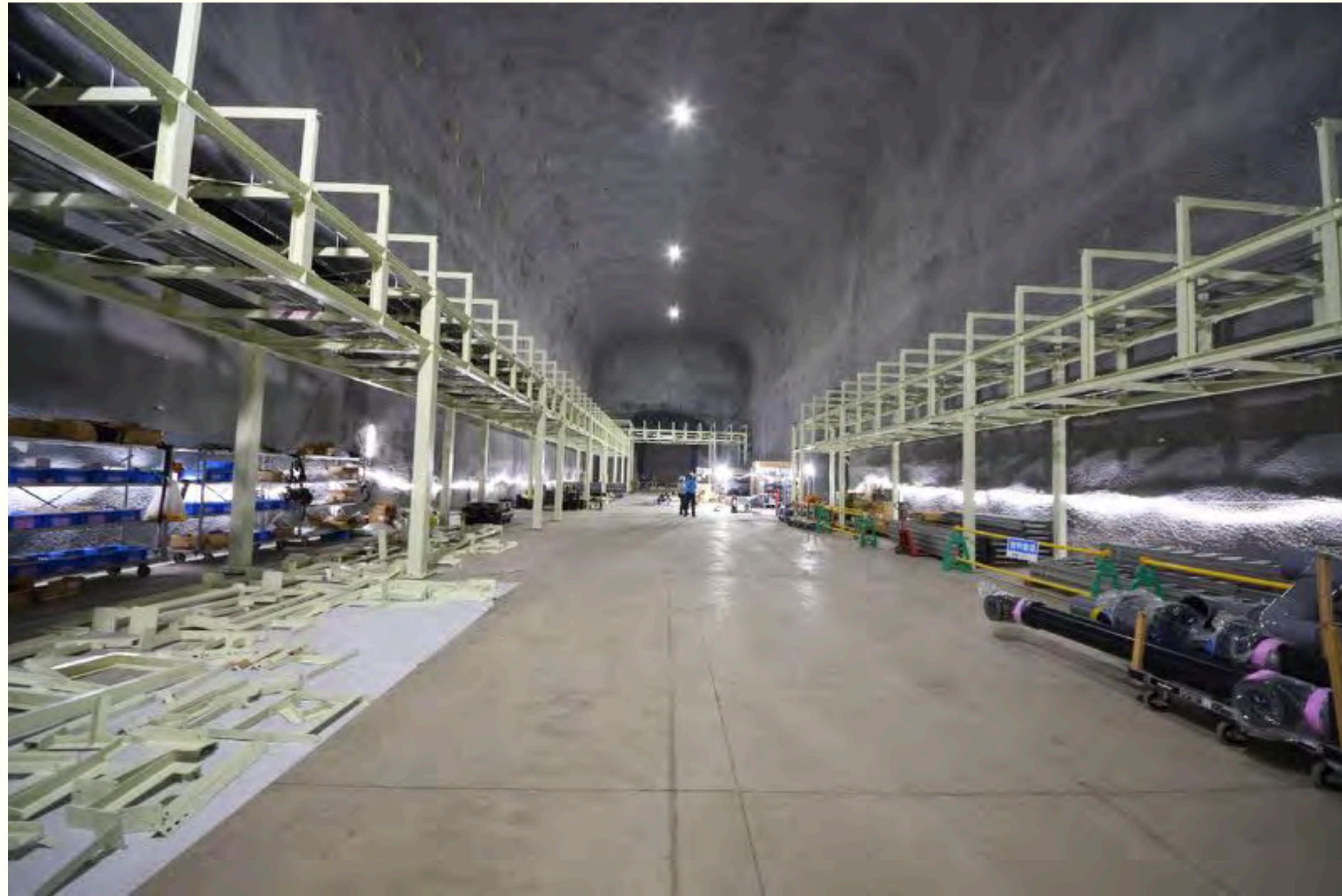
Water system room: ~half of Super-Kamiokande volume
